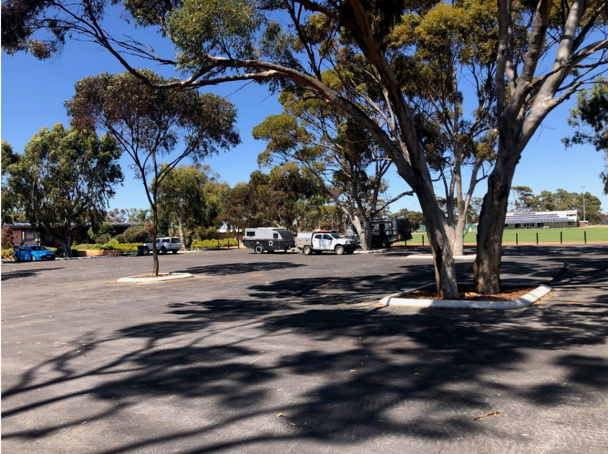
Hyden Swimming Pool sealed carpark
