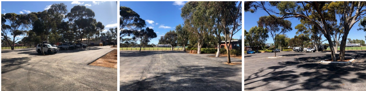
sealing Hyden and Districts Aquatic Centre carpark
