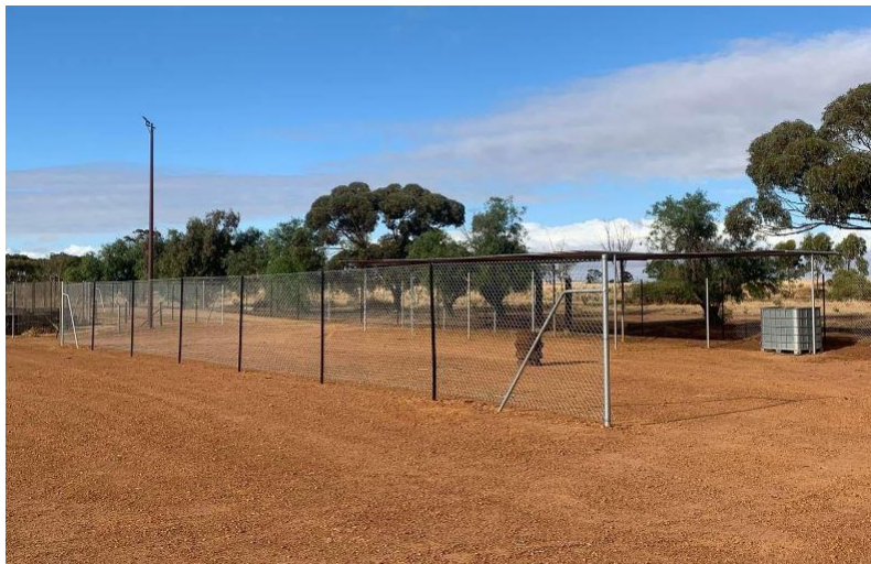
Kondinin Burnout Fencing Upgrade
